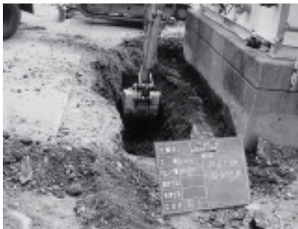
Removal of contaminated soil (former System Devices Division's Morioka Plant)
