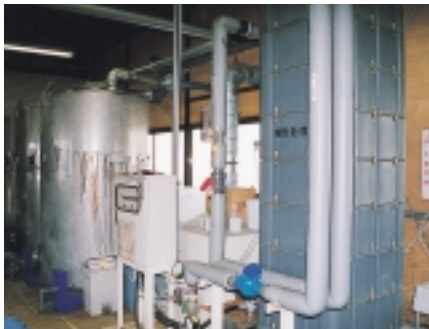
Groundwater treatment facility (Furukawa Plant)
