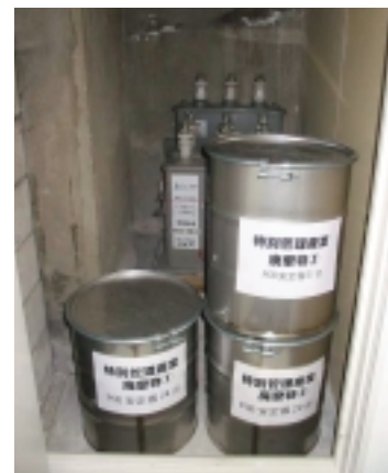
Storage facility for PCB (Headquarters)
