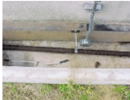
Above-ground pipes and oil leakage sensor (Peripheral Products Division's Onahama Plant)
