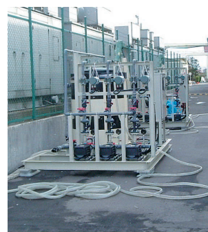
Nutrient injection equipment (Kakuda Plant)
