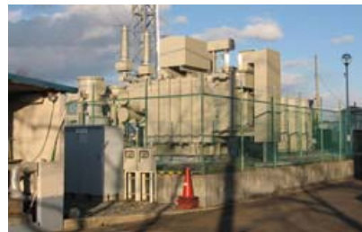
Extra-high voltage substation newly operated
