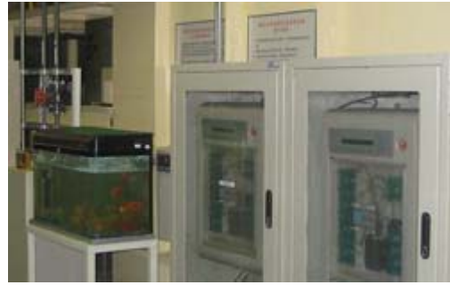
Wastewater discharge online system and raising goldfish with purified effluent.
