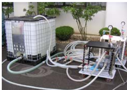
A device used in the past at Wakuya Plant (Miyagi Prefecture) to inject nutritional supplement into groundwater
