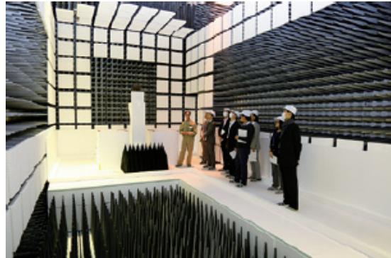
Plant tour for analysts (Furukawa Plant EMC Center)
