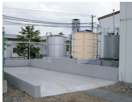
Chemical tank and leak reservoir (Furukawa Plant)
