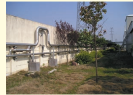
Wuxi Alps Electronics steam ducts
