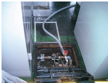
Nutrient injection well (Furukawa Plant)
