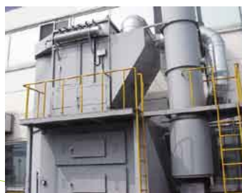
Active carbon tower to absorb VOCs (Alps Electric Korea)
